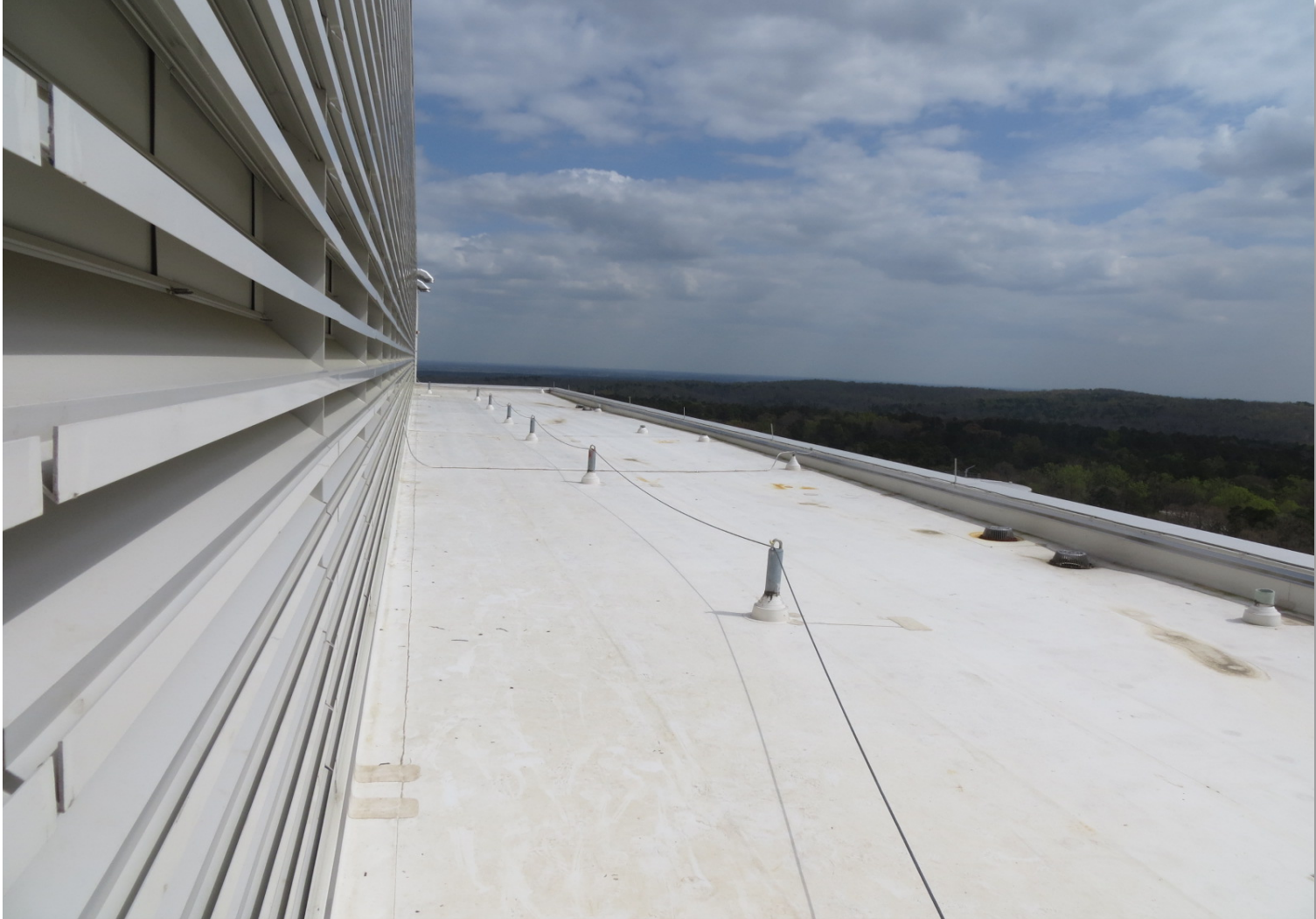
Marsico Hall – Energy Efficient Reflective Roof with Fall Protection
